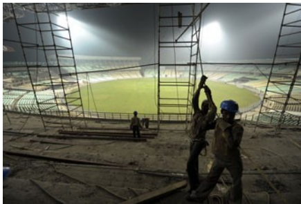
Construction has commenced on Phase 2.
